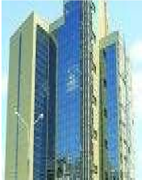
University IT Technological Park (under construction)
